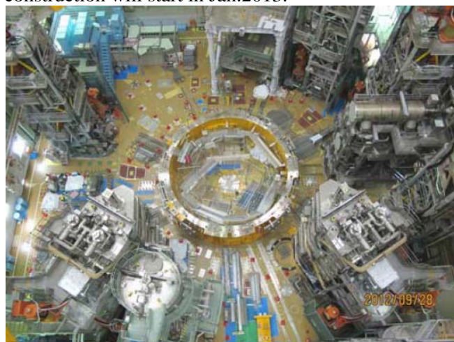
Fig.6 Disassembling of the JT-60 has almost been completed, and installation will start soon.
