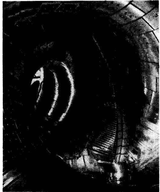
Fig. 2 A pair of ICRF heating antennas is installed at the higher magnetic field side on the outside of the torus in the LHD.
