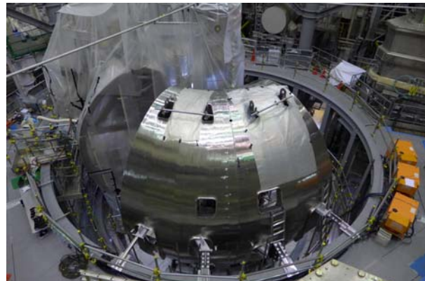
Fig.1. Welding Work of VV sectors in torus hall
