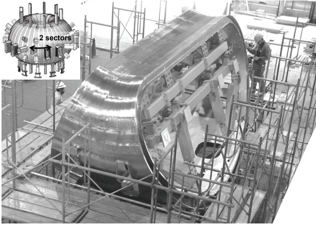
Fig. 2 First two sectors (40 deg.) of Vacuum Vessel was in the final inspection, and completed in May 2011 (left). characterized by the horizontal stiffness of 6.46 \times 10^2 MN/m and the design damping ratio of 5.0% at the plasma operational state. The welding technical elements are selected to validate its weldability and mechanical performance before product VV fabrication [7]. The product VV manufacturing is validated by these fundamental surveillance and several mock-up trials [5, 8].
