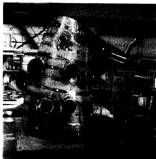
Fig. 3 Assembly of the plasma vessel (by courtesy of Balcke Dürr).
